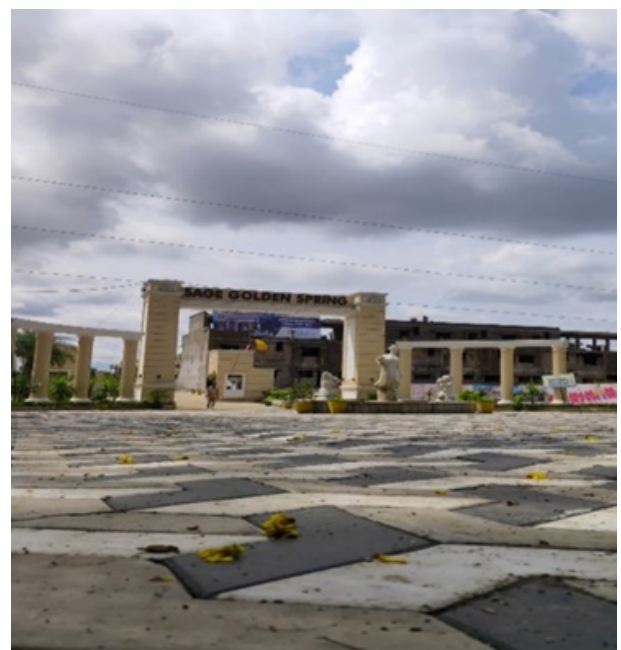
Figure 4: Project SGS site
