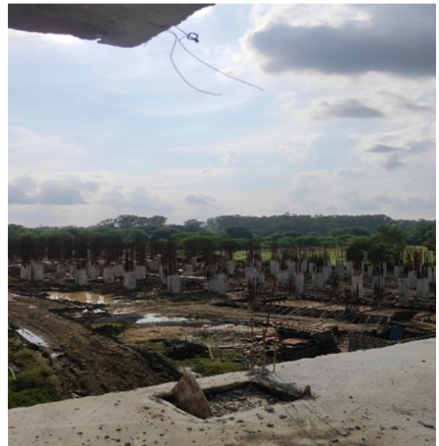
Figure 3: Top view of SGS site
