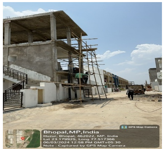
Figure 7: Project Suncity site
